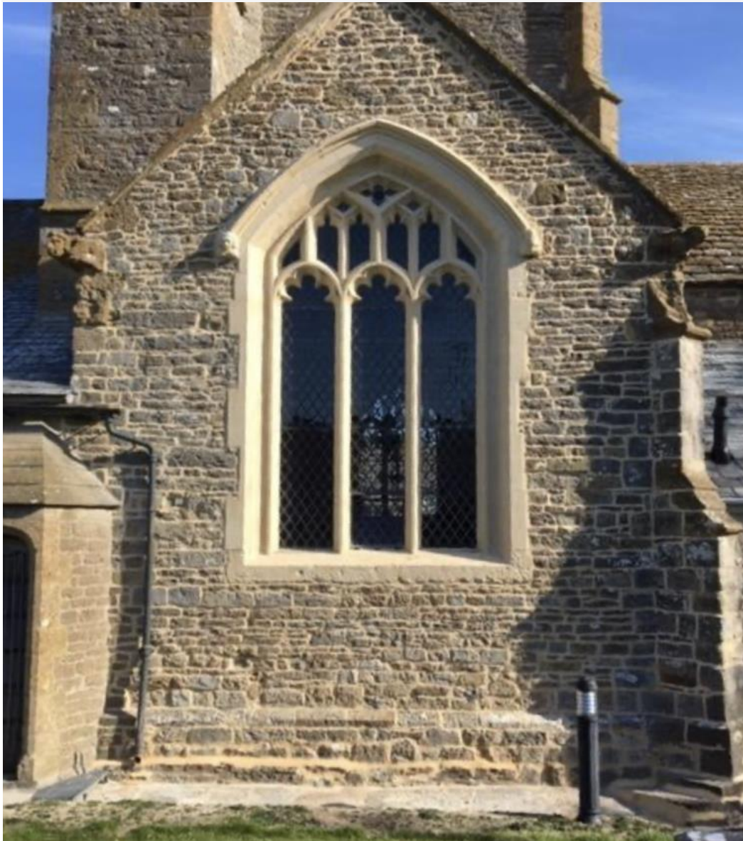
The new window at St Mary's Church, Burton Bradstock
